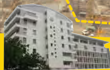
中學校舍地盤 Site of Secondary School
